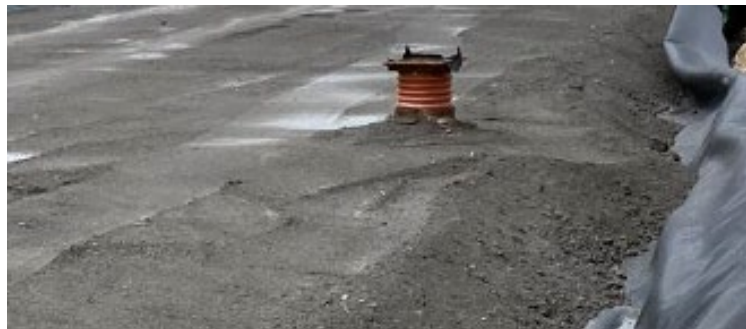
WtE IBA aggregate used as sub-base material in road construction
